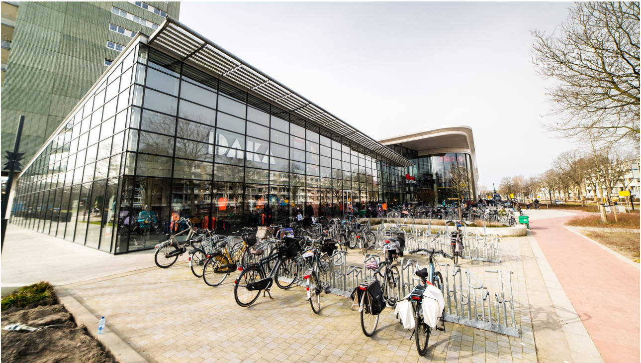
Figure 2: The construction of the Mall is based on the HUECK Trigon 50 façade system with integrated HUECK Lambda DS 075 door solutions (source: HUECK)
