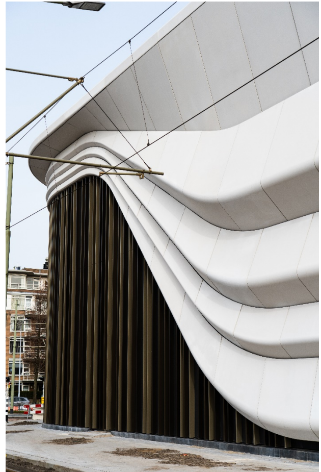
Figure 3: As with various preceding successful projects, TGM realized the extensive aluminium curtain wall with inserted aluminum with HUECK facade solutions (source: HUECK)
